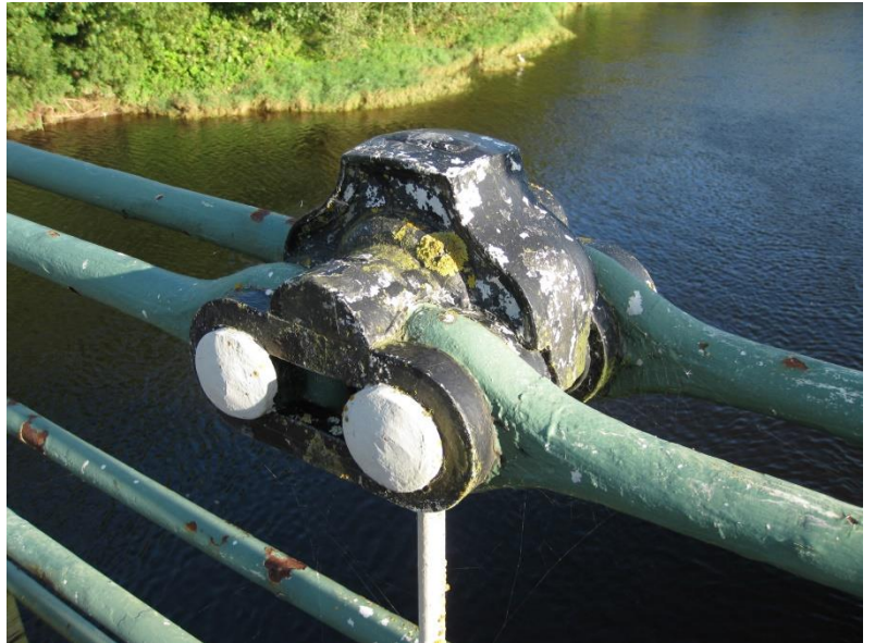
A chain link in the Union Bridge over the Tweed. This was the first chain link bridge to be opened in the world in 1820 connecting Scotland and England
